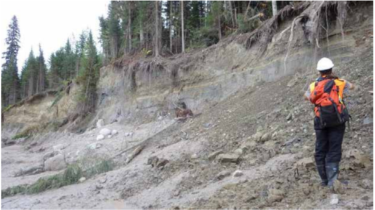
Photograph 15: View of ST09 area of scour exposing native parent mineral soil along exposed channel sidewalls (September 7, 2014).
