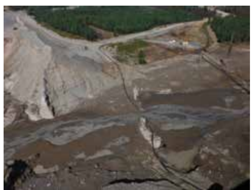
Aerial view of the TSF breach looking west. (September 05 2014)
