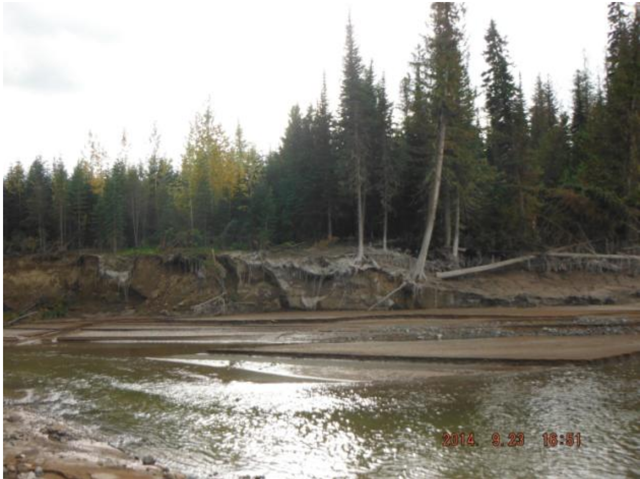
Figure 5-9: Photo shows slope failures at reach HC-R0b and red tailings deposited within the Hazeltine Creek channel (September 23, 2014).
