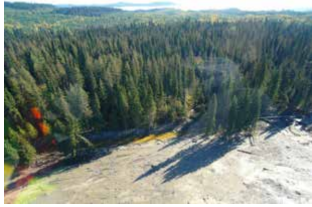
Eastern edge of plug area with nineteenth century diversion ditch (September 22, 2014).
