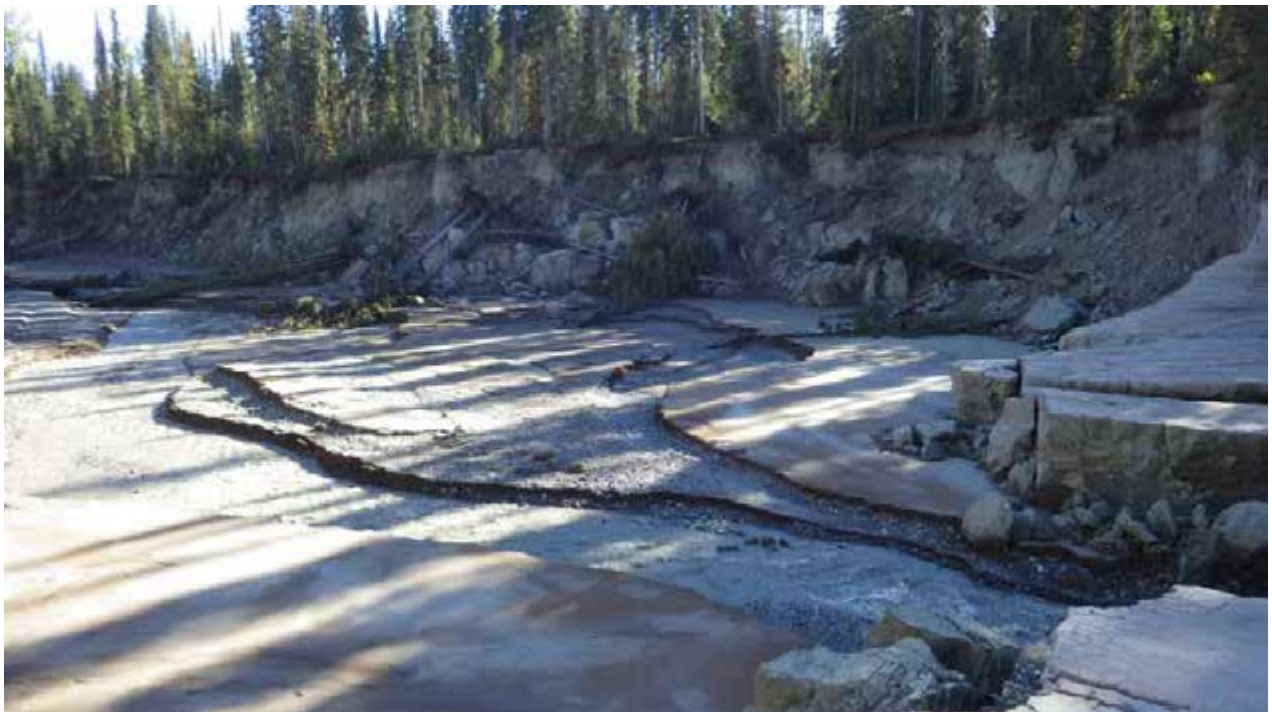
Photograph 4: View of ST11 showing unsafe access areas and unstable sidewalls (September 14, 2014).
