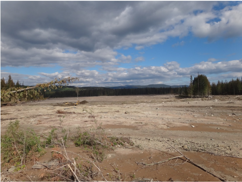
Photo 2. Eastward view from TMF breach.
