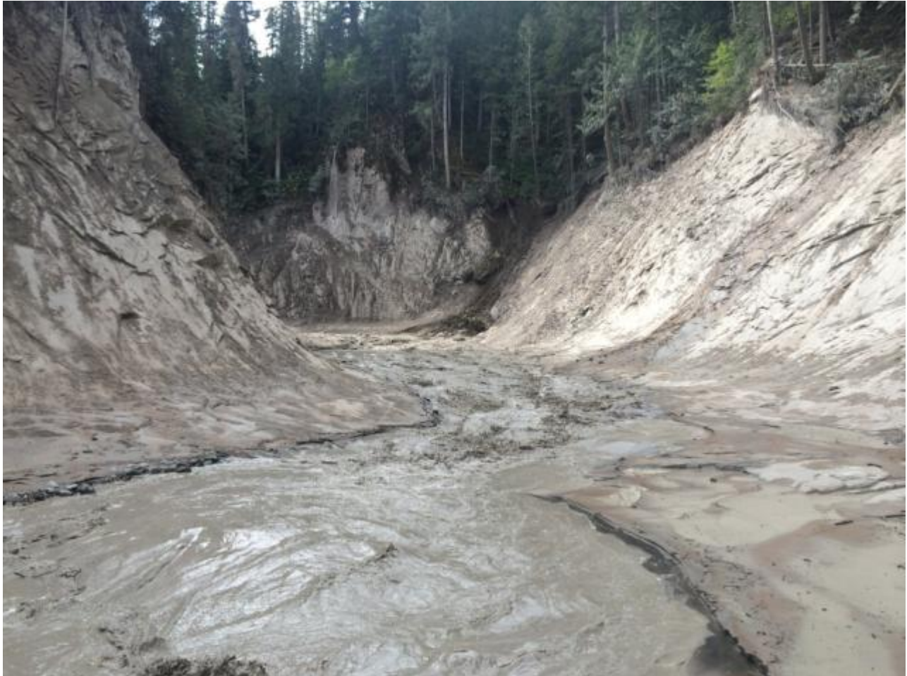
Figure 5-19: Photograph within the Hazeltine Creek Canyon showing exposed bedrock and a thin veneer of tailings at a wider section (HC-R6) looking upstream (August 26, 2014)
