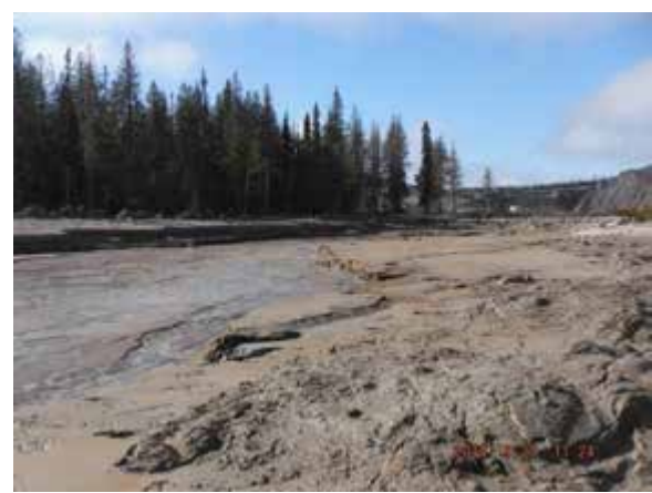
Upstream view toward the TSF. Flow from the TSF is incising into the native material and debris flow deposit (September 23, 2014).
