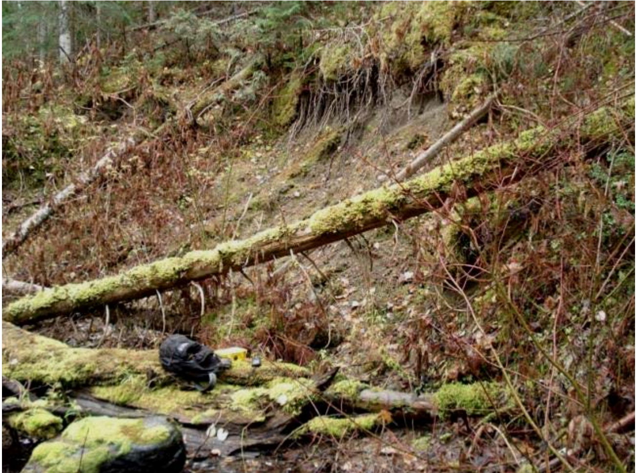
Figure 4-3: Bank failure in reach five of Hazeltine Creek. Photo from Minnow (January 20, 2007)
