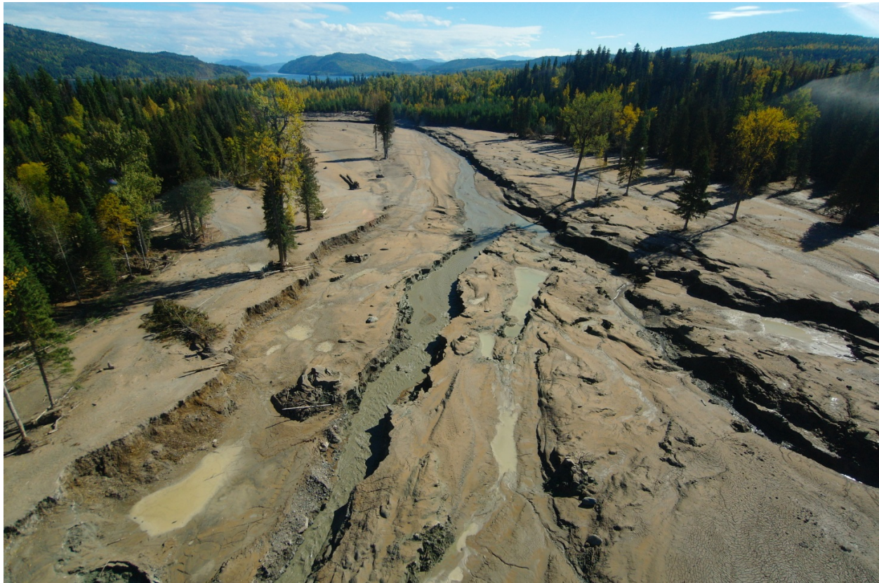
Figure 5-24: Reach HC-R8 looking downstream showing confluence of the debris flow bifurcation
