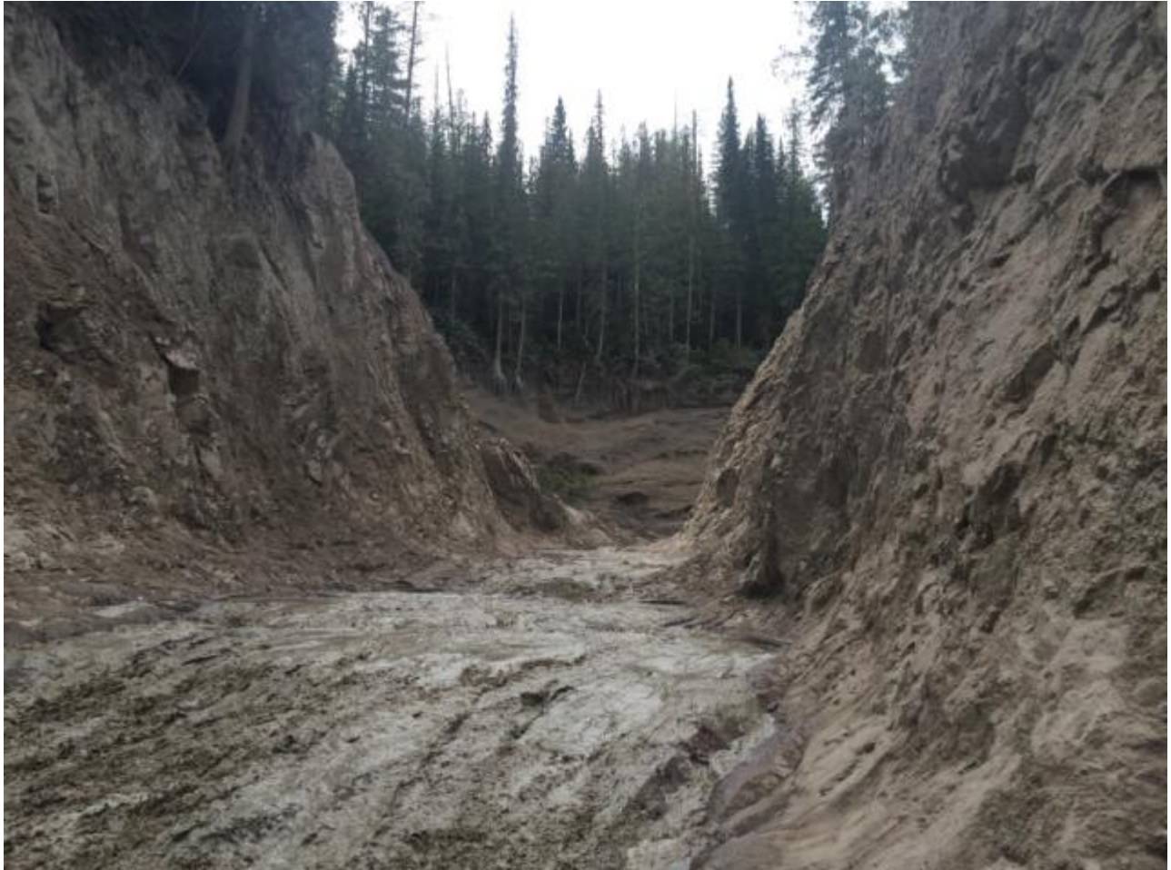
Figure 5-18: Photographs within the Hazeltine Creek Canyon showing exposed bedrock at a narrow section (HC-R6) looking upstream (August 26, 2014)
