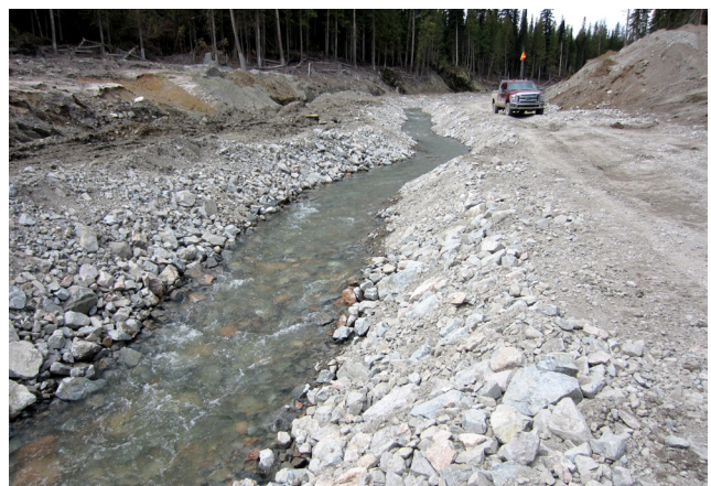
Photo 2: Mean Annual Flow channel construction
