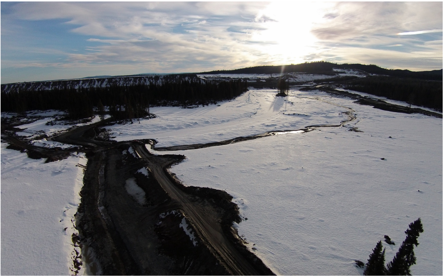
Reach 1 of Hazeltine Creek being constructed in the Polley Plug area
