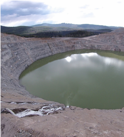
Mount Polley Mine diverted all site water collection systems to the Springer Pit
