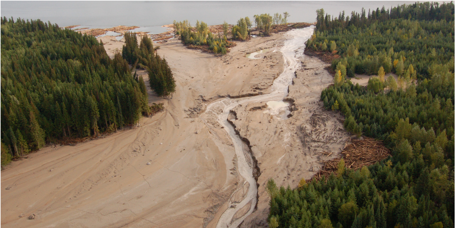
Lower Hazeltine Creek following the tailings dam failure (August, 2014) showing some of the physical changes that occurred
