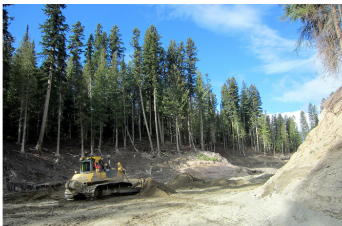
Photo 1: Floodplain grading
