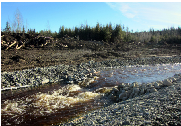
Photo 3: Construction of habitat features, including rock weirs, is underway
