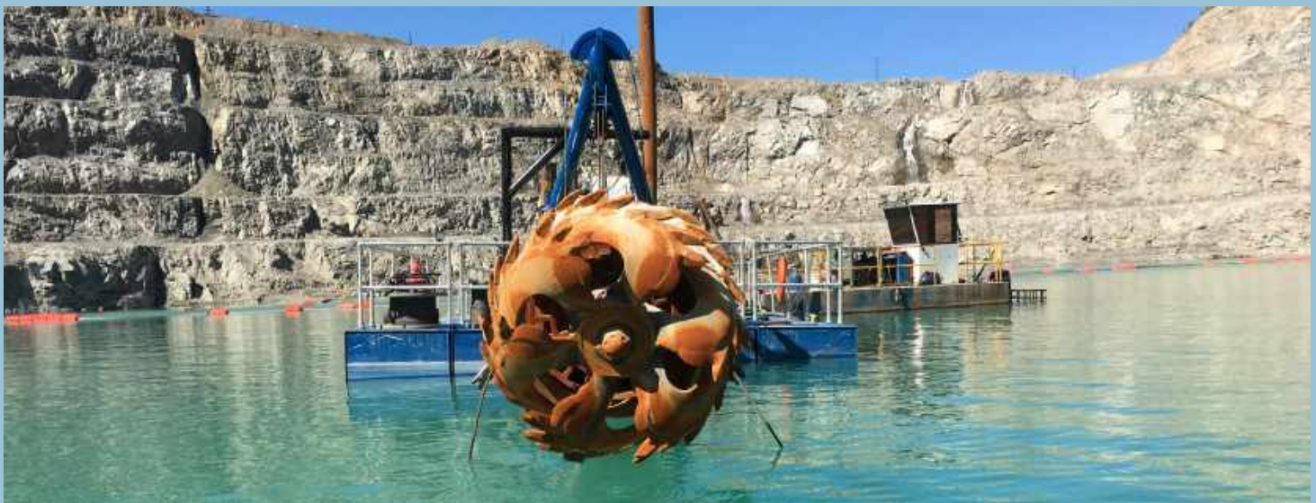
The cutting head for the dredge is used to cut and agitate the materials before being sucked into the dredge and pumped to the TSF.
